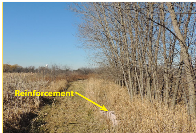
View north along berm. Low point on berm reinforced at seasonal outlet from CMA into WMA.
